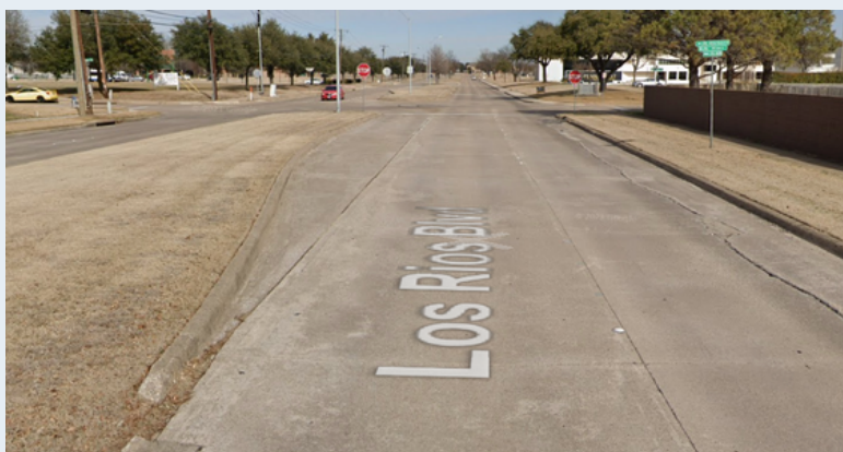
Figure 5. Northbound on Los Rios Boulevard at Merriman Drive- The City of Plano Transportation Division identified missing advanced warning Stop Ahead (W3-1) signs at all four approaches. Per MUTCD Table 2C-4 for a 35 mph condition, the Stop Ahead (W3-1) sign shall be placed 100 feet in advance of the Stop (R1-1) sign.
