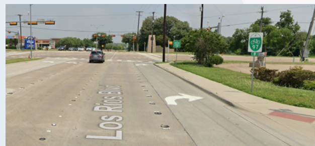
Figure: 6. Los Rios Boulevard and 14th Street- The City of Plano Transportation Division identified missing mandatory movement lane control signs, i.e. Right Lane Must Turn Right (R3-7) and Right Turn Only (R3-5) signs.
