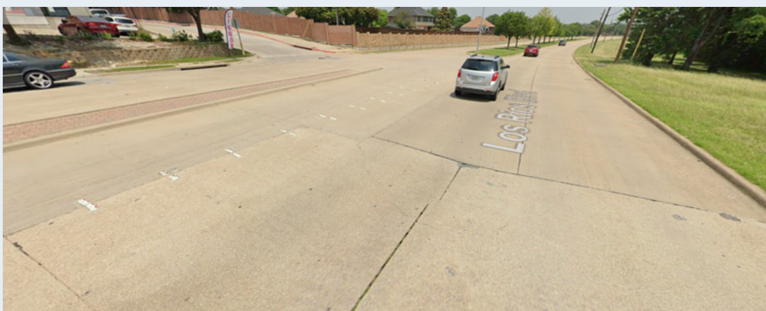
Figure 8. Abrupt lane drop traveling northbound on Los Rios Boulevard at 14th Street
